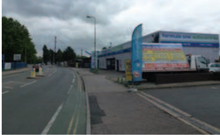
Light industrial unit fronting Oxpens Road
